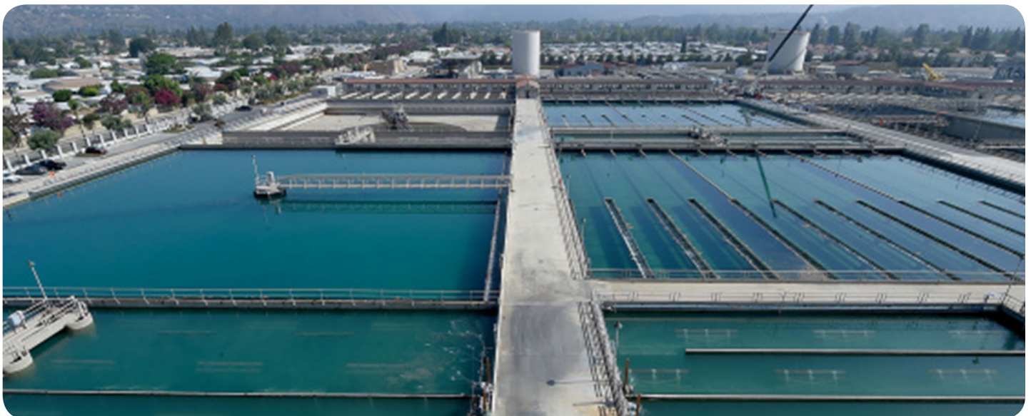
This image shows one of Southern California's water treatment facilities, which filters contaminants before water reaches our taps. Photo credit: The Metropolitan Water District of Southern California.
